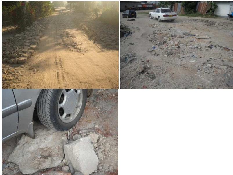
Figure 4. The reuse of concrete rubble for filling pothole in Dar es Salaam (taken Ukonga and Mwenge, 20010)
