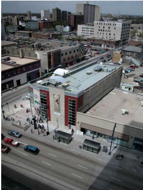
Left: A C-2000 Demonstration project in Winnipeg, Canada, in which 95% of the materials of two existing materials were incorporated in the new building. This project, which featured 50% better energy performance than conventional buildings created a high level of interest in the whole region, at comparatively modest cost.
