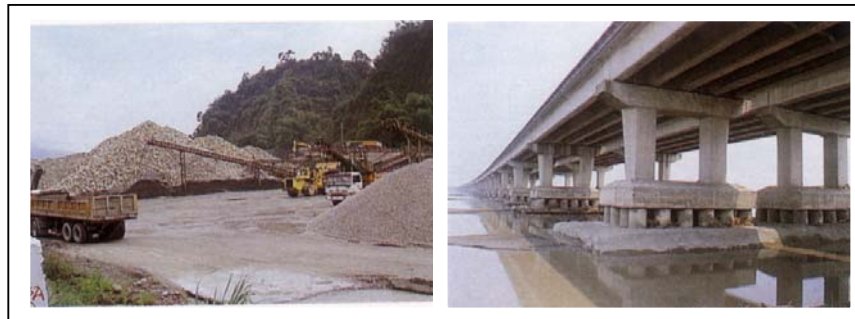
Fig.1 Illegal Aggregate Excavation is detrimental to bridge safety
