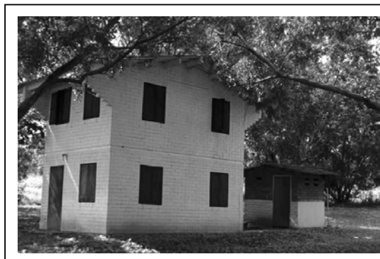
Fig.4 A soil/cement prototype house built at the Asian Institute of Technology in Bangkok
