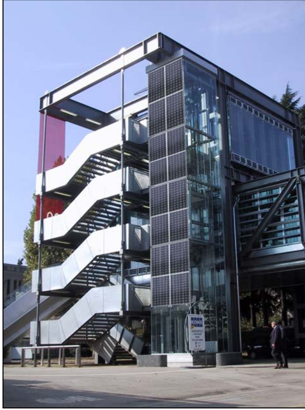
Fig.2 The PV installation under development in Italy
