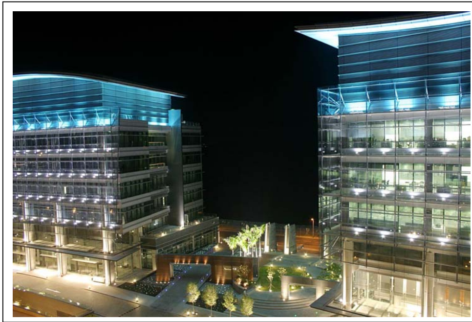
Fig.7 Night view of courtyard and buildings
