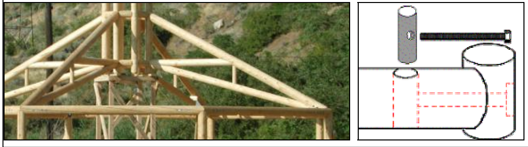
Fig.1 Round wood trusses ( www.fpl.fs.fed.us )
