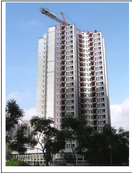
Fig.12 Progress photos of building
