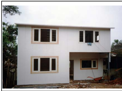
Fig.6 Front view before wood siding
