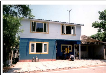
Fig.7 Front view after completion Site
