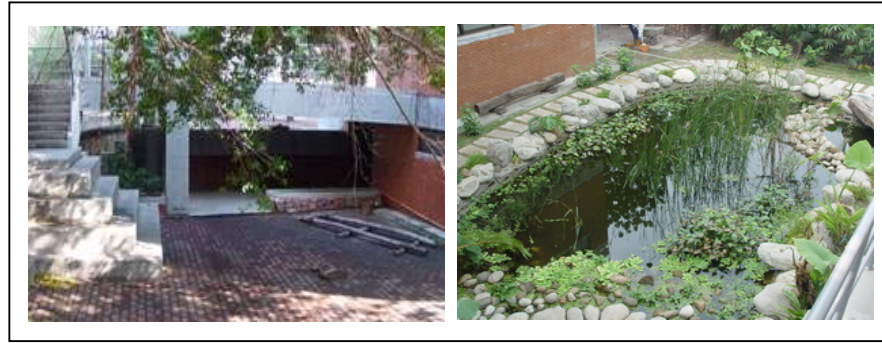
Fig.5 Green Remodeling Project – constructed wetland (ABRI, 2004)
