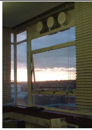
Fig.3 Existing glazing with steel framing
