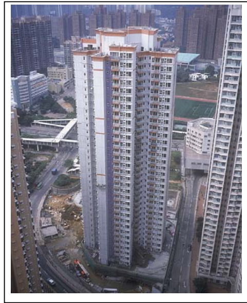
Fig.13 Completed building elevation
