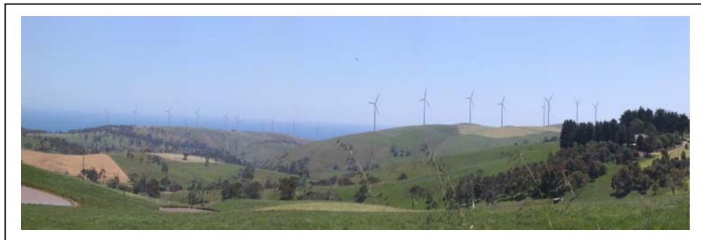
Fig.2 Starfish Hill wind turbines, near Cape Jervis, Fleurieu Peninsula, South Australia
