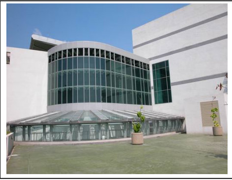
Fig.2. The Thermal flue stack to generate natural ventilation in the atrium
