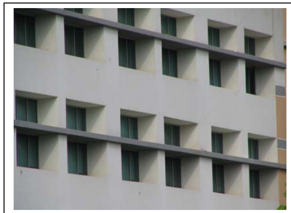
Fig.4 The "Punch Hole" windows provide shading to the windows
