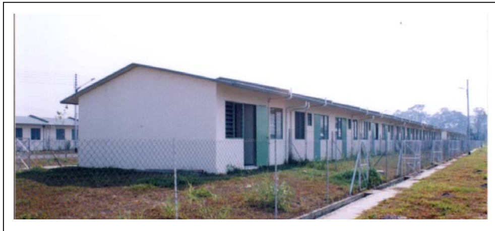
Fig.1 Low-income housing located in Kuching, Sarawak
