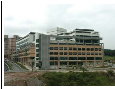
Fig.1 The East Façade of the LEO Building
