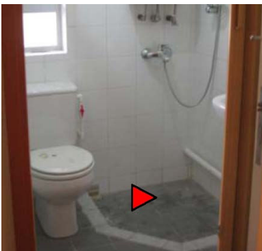
Figure 10 Sunken Shower with Installation of Grating by Tenants
