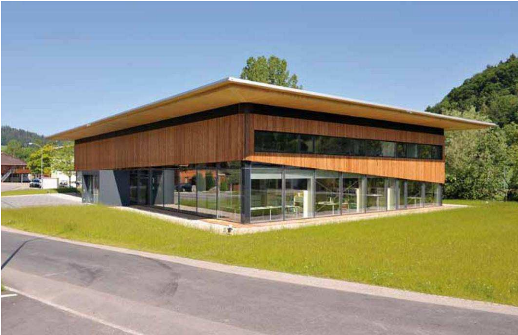
Fig. 1: MINERGIE-ECO-certified building (administration building company Zaugg, Rohrbach, Canton Bern)
