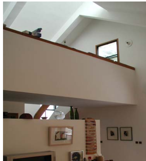
Fig. 1. Shaviv House - A Passive Solar Residential Building: Example of solar retrofit of existing building located in a high density urban area [7]. The passive system is a "Central Window Sunspace System (CWSS)" that collects the solar radiation at the roof top and transfers it to the first floor that is shaded by its neighbouring building. The CWSS serves also as wind chimney and thermal chimney that ensuring natural ventilation in the building (Arch. Edna Shaviv).
