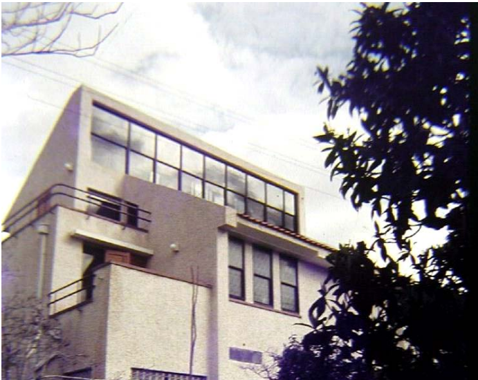
Fig. 1. Shaviv House - A Passive Solar Residential Building: Example of solar retrofit of existing building located in a high density urban area [7]. The passive system is a "Central Window Sunspace System (CWSS)" that collects the solar radiation at the roof top and transfers it to the first floor that is shaded by its neighbouring building. The CWSS serves also as wind chimney and thermal chimney that ensuring natural ventilation in the building (Arch. Edna Shaviv).
