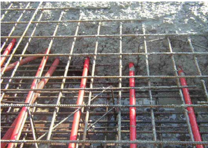
Fig. 6 Fabrication of thermo-active concrete slab (on site)
