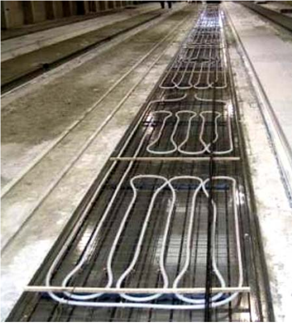
Fig. 7 Fabrication of thermo-active hollow-core slab (in shop)
