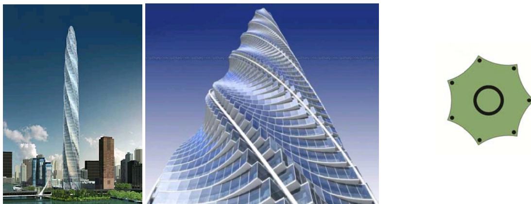
Fig. 2 Chicago Spire, Chicago, USA (source: Chicago Spire LLC) and its floor plan
