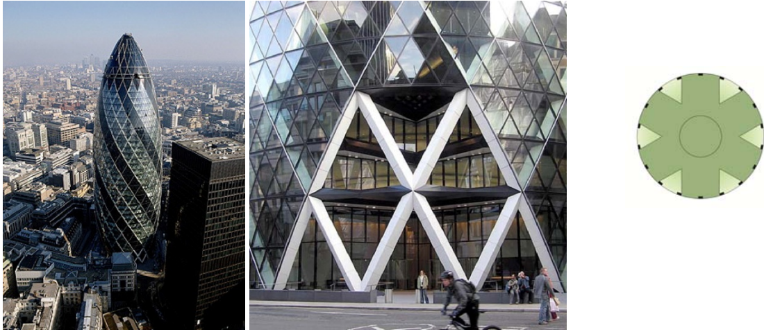
Fig. 6 Swiss Re Tower, London, UK (source: Foster and Partners) and its floor plan
