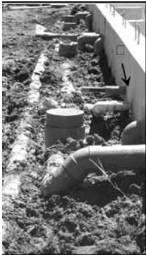
Photo. 5 – Successively placed small-size catch basins drainage pipes, have been developed.
