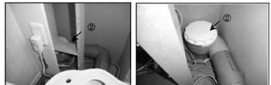
Photo. 3 – Stack-horizontal branch merging section
