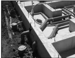
Photo. 6 – Pass-through section of the foundations
