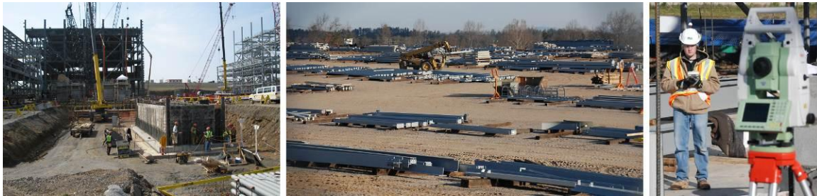
Figure 3: Layout of experiments: Construction pit (left), lay down yard (middle), and UWB tag and RTS prism on helmet (right).
