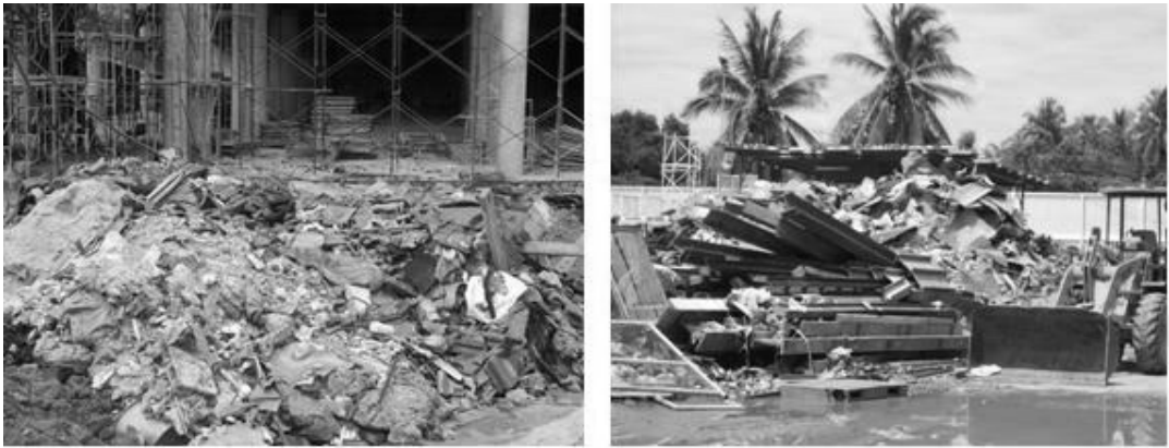
Figure 2: Mixed and improper store of C&D waste
