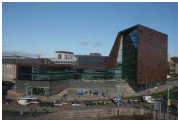
Figure 4: Photo of the Roland Levinsky Building at the University of Plymouth campus
