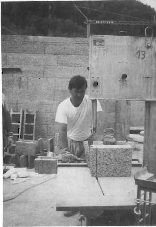
Figure 4. Cutting wood-cement with regular band-saw.
