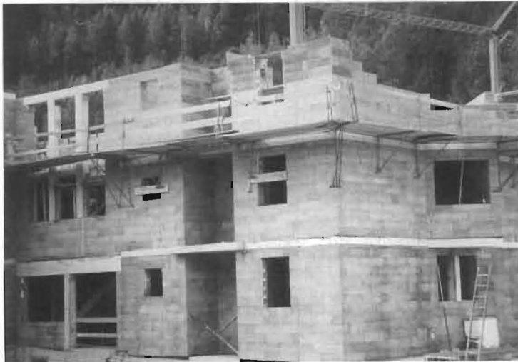
Figure 3. Condominium project built with wood-cement stay-in-place insulated forms
