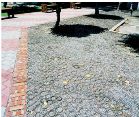
Figure 4 Permeable pavement in Tai-Tung Vocational School (Source: ABRI, 2006)
