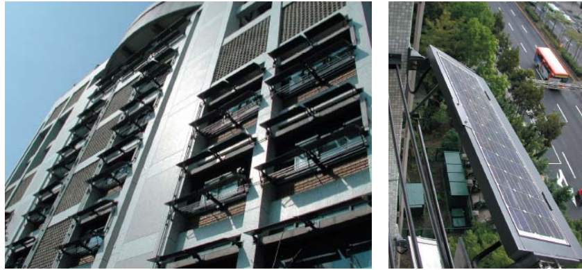
Figure 5 Installation of outer sun-shading incorporating with solar cell system (Source: ABRI, 2004)
