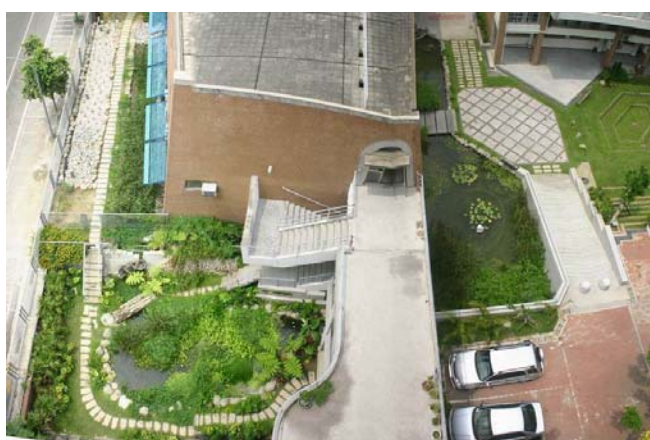
Figure 2 The constructed wetland in the National Cheng Kung University plays a demonstrative role in environmental education (Source: Jui-Ling Chen, 2005)
