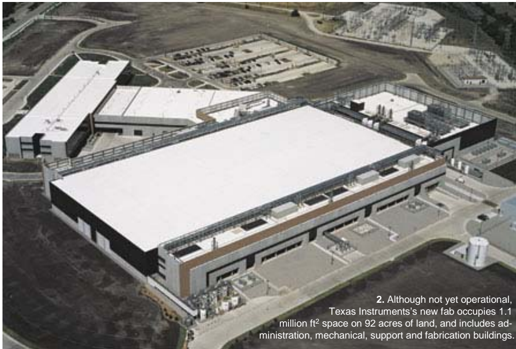
Fig. 3 TI RFAB, the 1 st LEED Gold Rating FAB (Semiconductor International, 12/2007)
