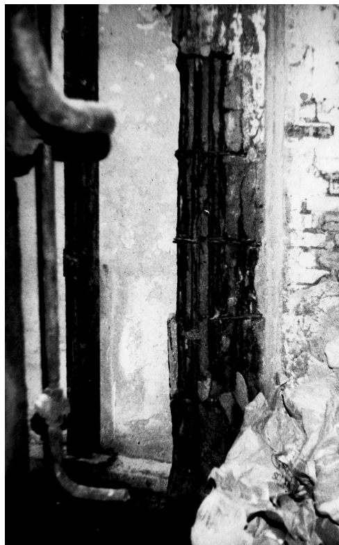
Fig.1. One of columns in emergency condition
