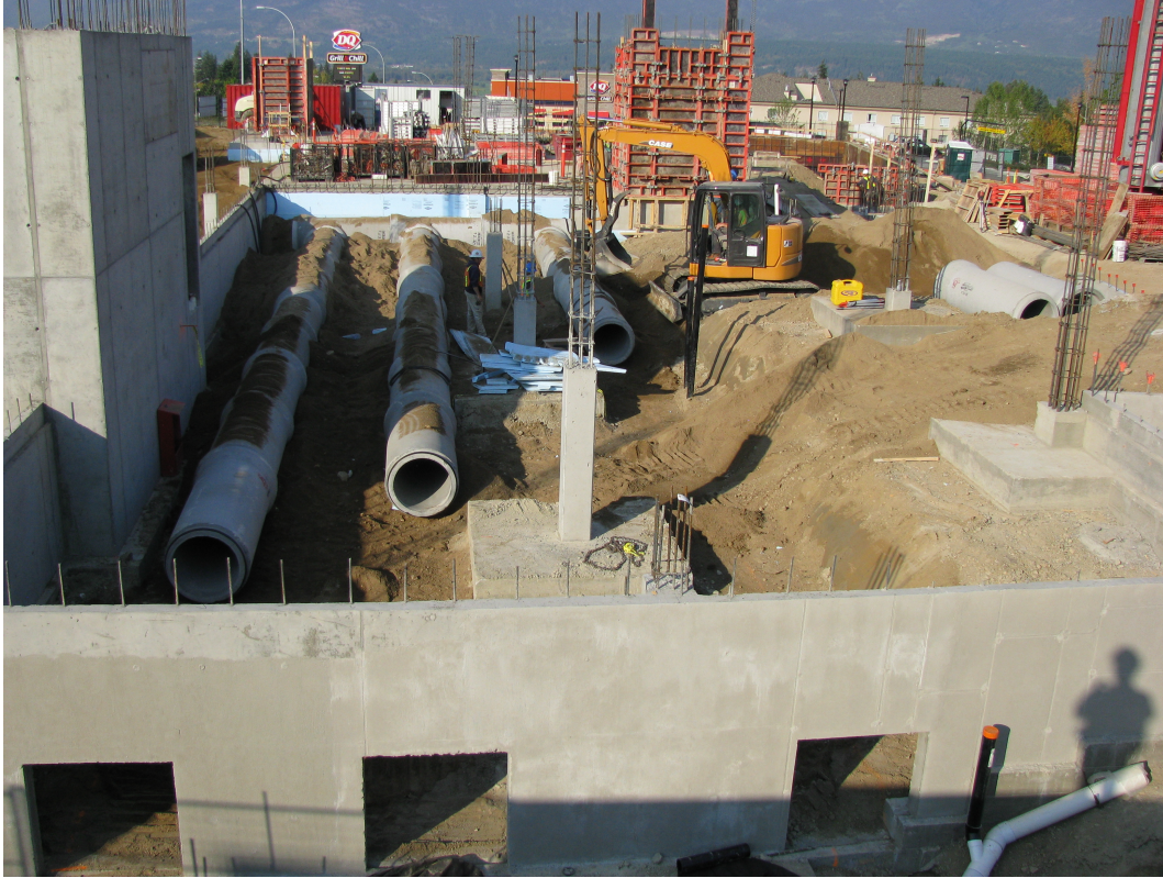
Figure 1. SASCU earth tube system under construction, 2012.
