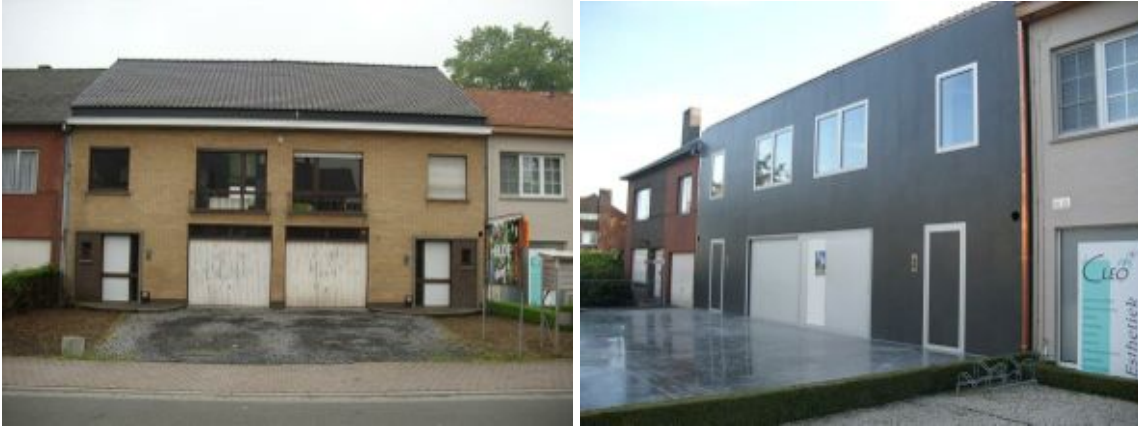
Fig. 1: Retrofit of 2 row houses from the 1970s. Before (left) and after (right) © Benergie.be – Architect L. Dedeyne
