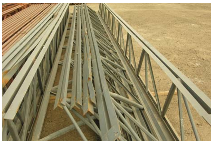
Figure 1: Open web steel joists can often be dismantled for reuse, but the new structure needs to be based on the available spans
