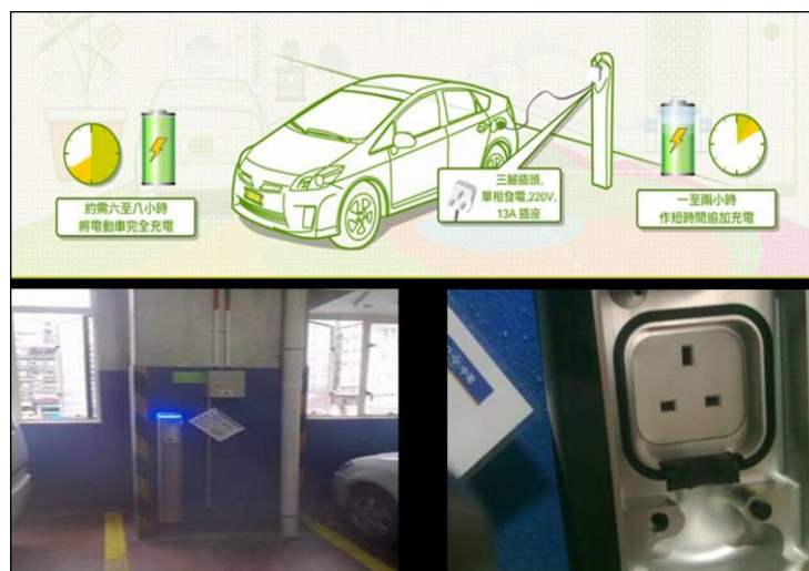
Figure 7: Charging Facilities for Electric Vehicles
