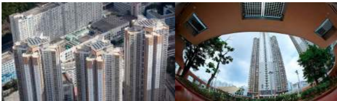
Figure 3 PV panels installed on the upper roof for the maximum solar absorption (left), PV panels installed over the pedestrian level to enhance awareness on the use of solar energy to the building users. (right)
