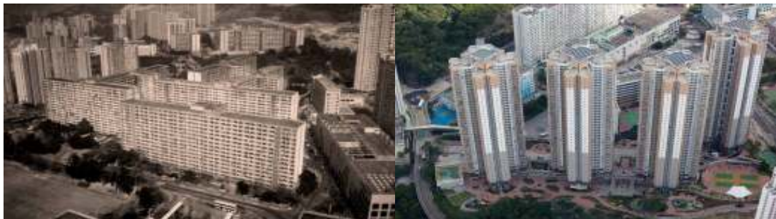
Figure 1 Old Lam Tin Estate (left) New Lam Tin Estate (right)
