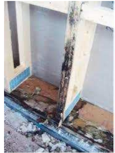
Fig 2.3 Moisture damage
