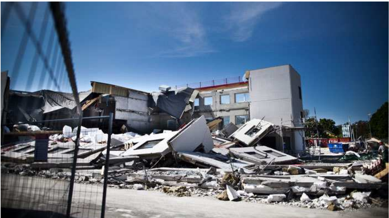
Fig 2.1 Building in Ystad collapsing two weeks before inauguration as “the House of Health”
