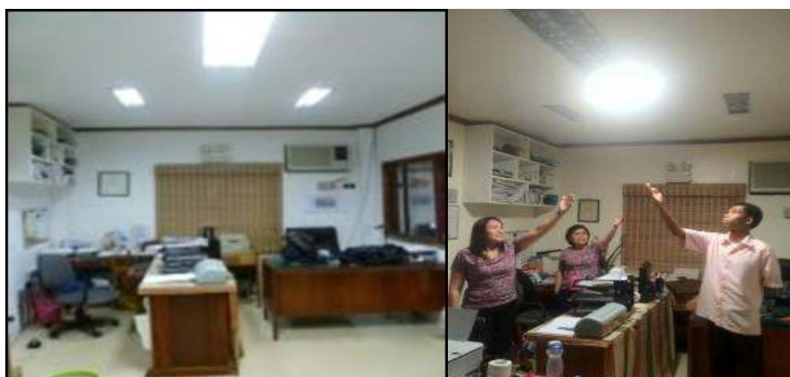
Figure 8 Installation of tubular solar lighting
