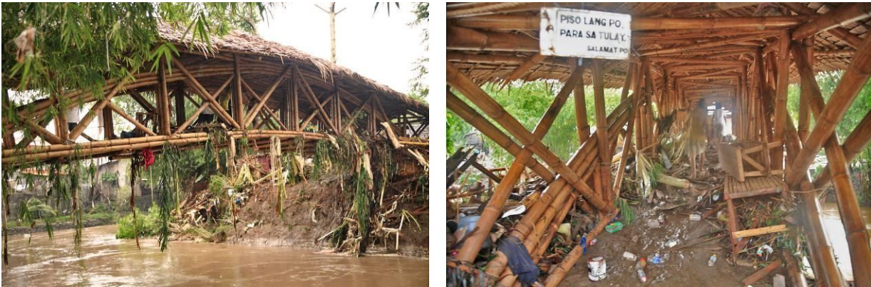
Figure 10 Debris brought by July 27 flash flood (left) engulfed the bridge (right), and the concrete floor which seamlessly connects the bridge to its foundation saves the bridge.
