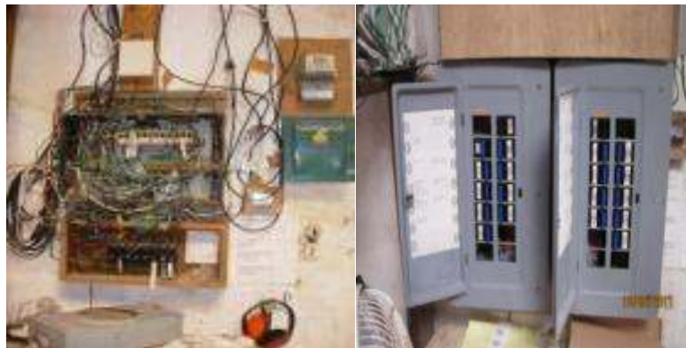
Figure 5 (before) Unorganized electrical wiring system may cause danger (after) Organized and labelled electrical wiring system
