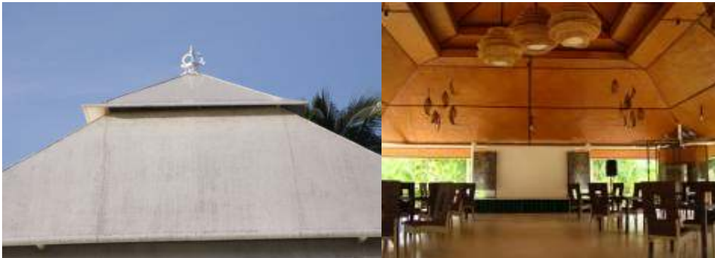
Figure 10 After: Improved pavilion with installed water sprinkler, insulation at the roof, wooden ceiling and rattan chandelier for better aesthetic effect and as an added insulation
