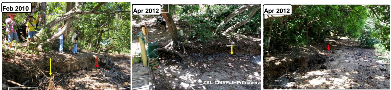
Figure 13 Backshore elevation before and after breakwater construction (ZSL-CMRP photos by J.H. Primavera)
