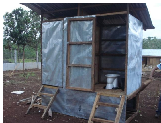
Figure 7 Ecosan Toilet in CDO Resettlement Site
