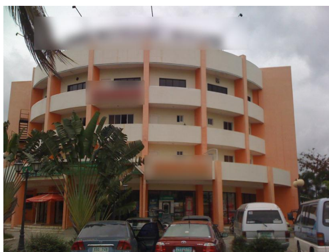
Figure 68 Facade of Hospital C
