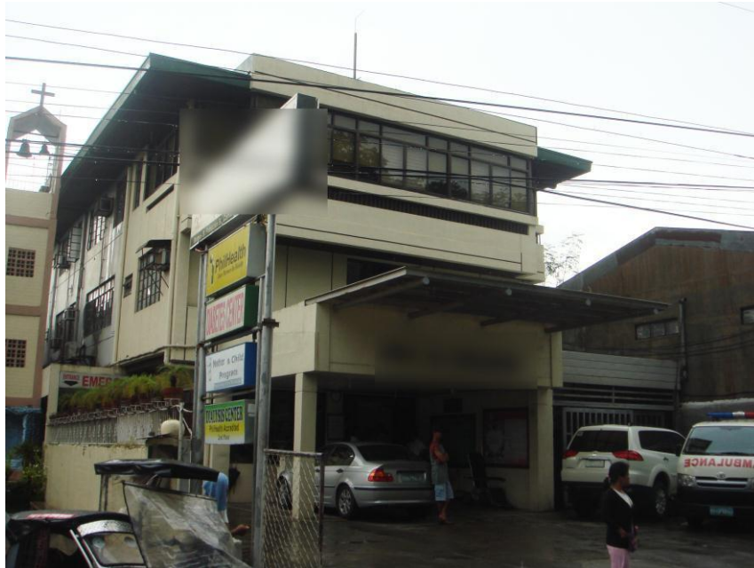
Figure 62 Facade of Hospital A
