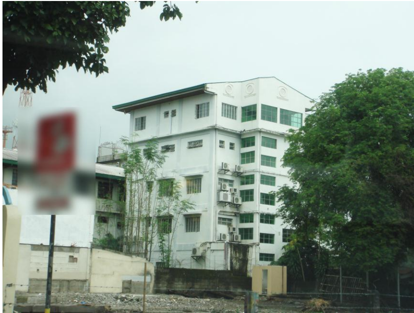
Figure 63 Hospital A Annex Building
