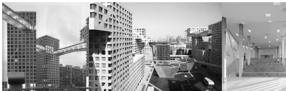
Figure 04 (left to right): The Linked Hybrid , Beijing: skycourts, skygardens and skybridges seek to reduce perceived densities
