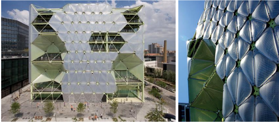
Figure 3: Smart envelope comprised of ETFE encased solar-activated lamella shades developed for the Media-TIC building in Barcelona, Cloud 9 Architects 2011 (Source: Addington and Schodek, 2010)
