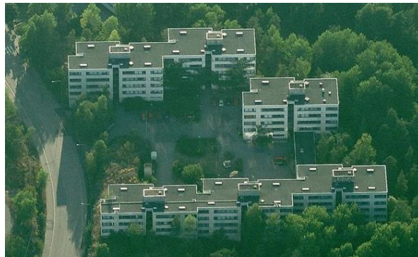
Fig. 1: Property overview prior to the start of the construction project.
