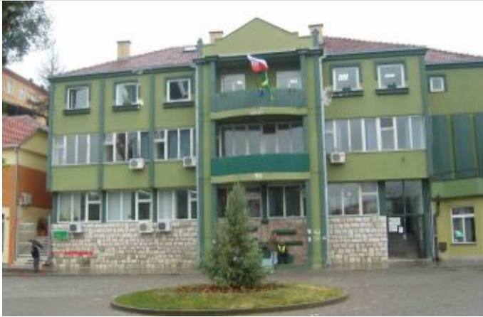
Fig. 3: Case study building
