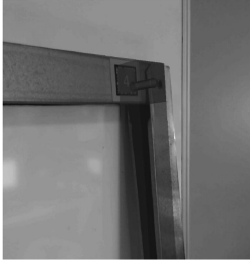
Figure 6: Truss with incorrect AR alignment
