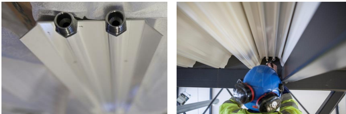
Figure 4: Ruukki radiant profile and installation
