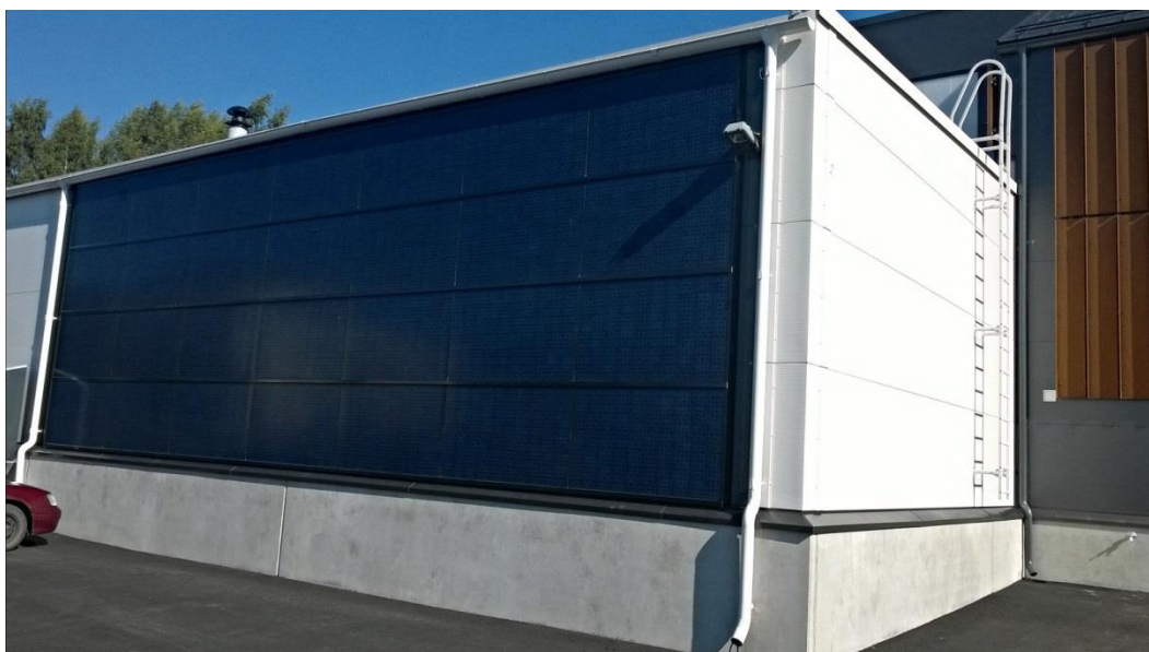
Figure. 9: Building-integrated solar PV panels installed on the southern facade
