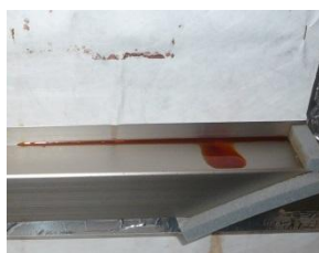
(a) Lye on the flashing
