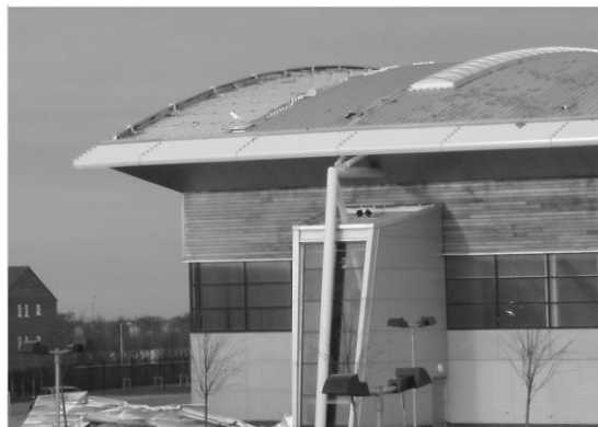
Figure 2: Detachment of aluminium standing seam roofing from windward verge
