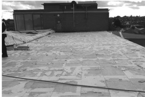
Figure 4: Roof membrane rolled back from western edge
