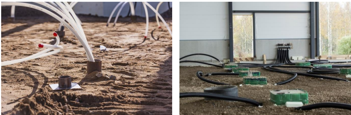
Figure 6: Heat collector pipes installed in the floor slab piles
