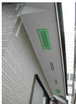
Photo 1—Eaves vent of the experimental house (north side).
