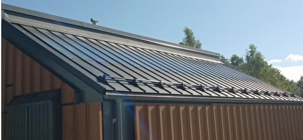
Figure 7: Roof-integrated solar heat collectors
