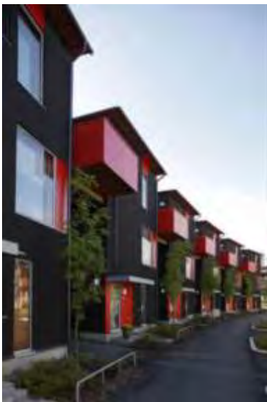
Fig 5. The building fulfills the requirement for visitability, but not accessibility (Helsingin Huvitus, ATT)
