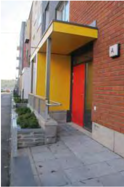
Fig. 3. A narrow front yard ensures privacy and allows construction of an accessible entrance. The platform before entrance is too narrow for wheelchair use or mechanical removal of snow. (Kalasatama, Helsinki).
