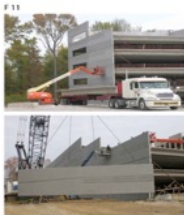
Description: Precast concrete panel system for a car park Source: WMU, Center for Weather and Climate Prediction, University of Maryland
