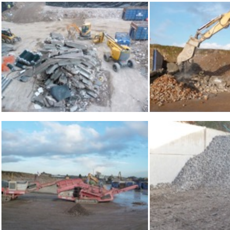
Figure 7 Stages of concrete demolition and recycling with the potential to cause dust release
