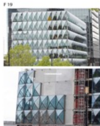
Description: Mixed concrete and glass panel facade system Source: (inter concrete system covered by glass panels) courtesy of the School of Property, Construction, and Project Management at WMU University
