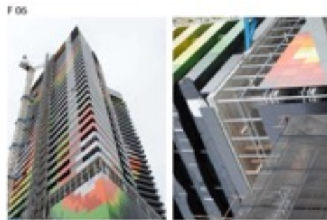
Description: Mixed metal/glazed panel facade system Source: courtesy of the School of Property, Construction, and Project Management at WMU University
