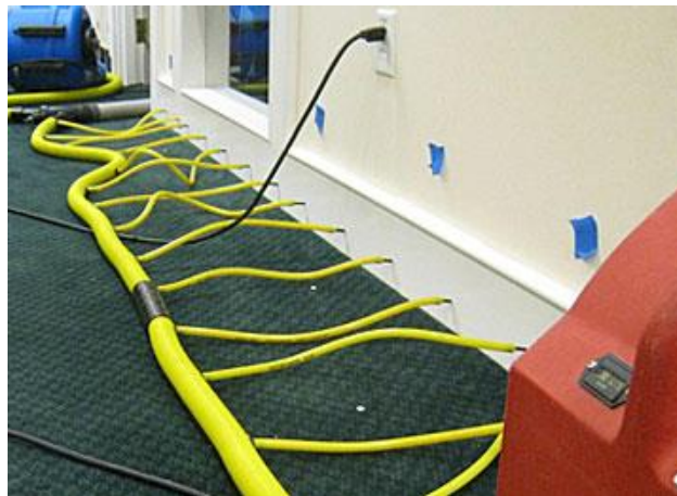
Figure 5: Drying wet wall with presence of insulation
