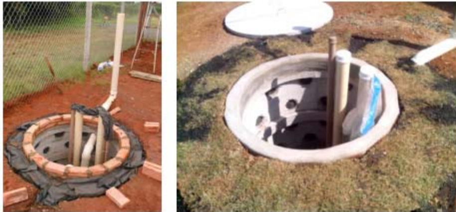
Figure 1 Stormwater infiltration dry-well [6]
