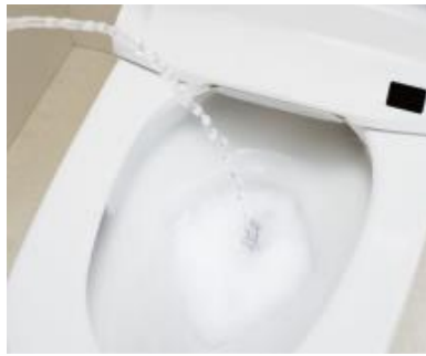
Figure 1 A picture showing passing urine towards foam supplied to a toilet bowl
