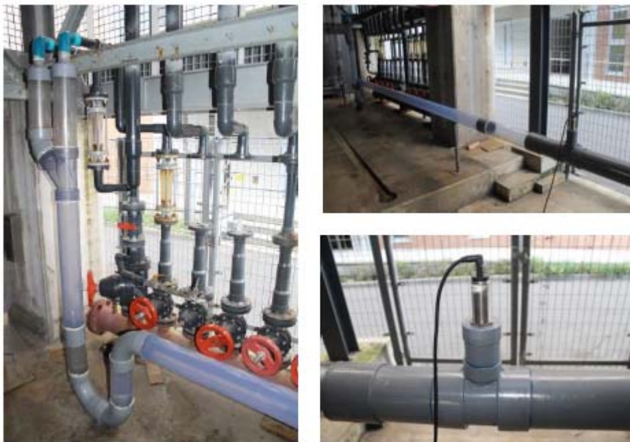
Photo 2 Experimental horizontal drainpipe system in the laboratory
