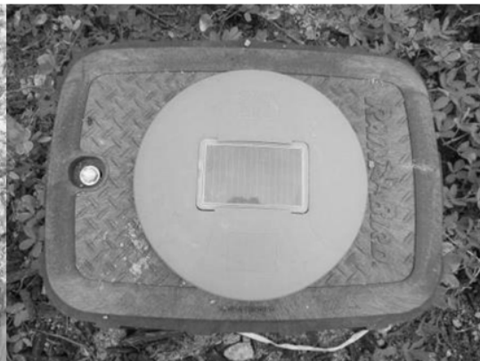
Figure-23 Solar powered solenoid vaive-solar cell
