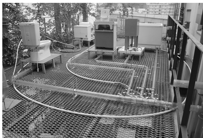
Fig. 8 Experimental horizontal drain branch system
