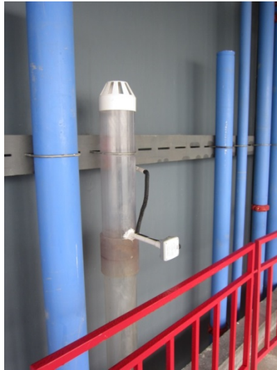
Fig. 3 Installation photo of the anemometer
