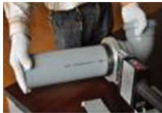
Fig. 3 After hot melt socket connection
