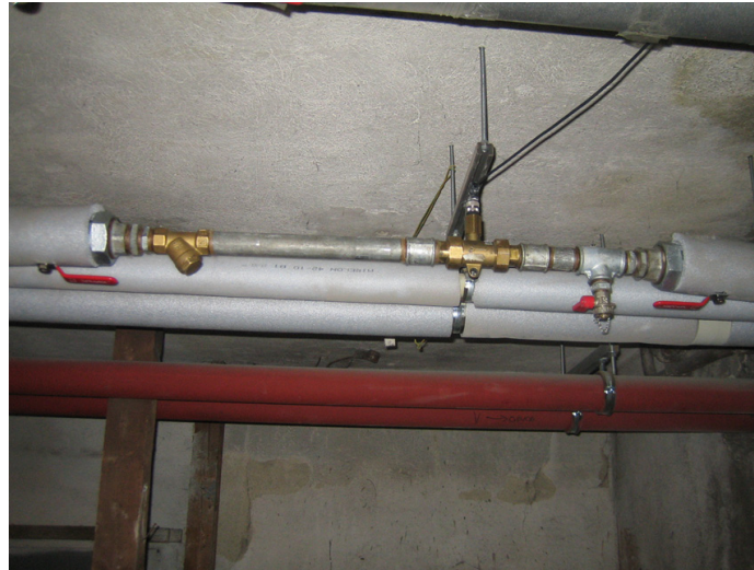
Figure 6 - Location of flow meters in residential building
