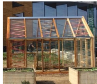
Figure 6. Tivoli – greenhouse of Tomato Chili made of reclaimed wood and glass
