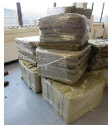
Figure 4. Horta-ONSS – repackaging of insulation for off-site reuse.
