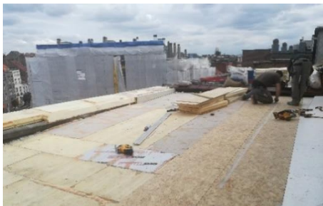
Figure 5. Petite Suisse – roof insulation made with over-ordered insulation boards from Debatty project
