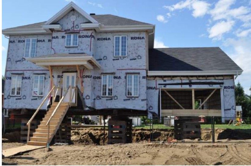
Figure 1: Replacement of the concrete foundation. All the masonry and covering stones were removed, houses were lifted up and concrete foundations were demolished and replaced.
