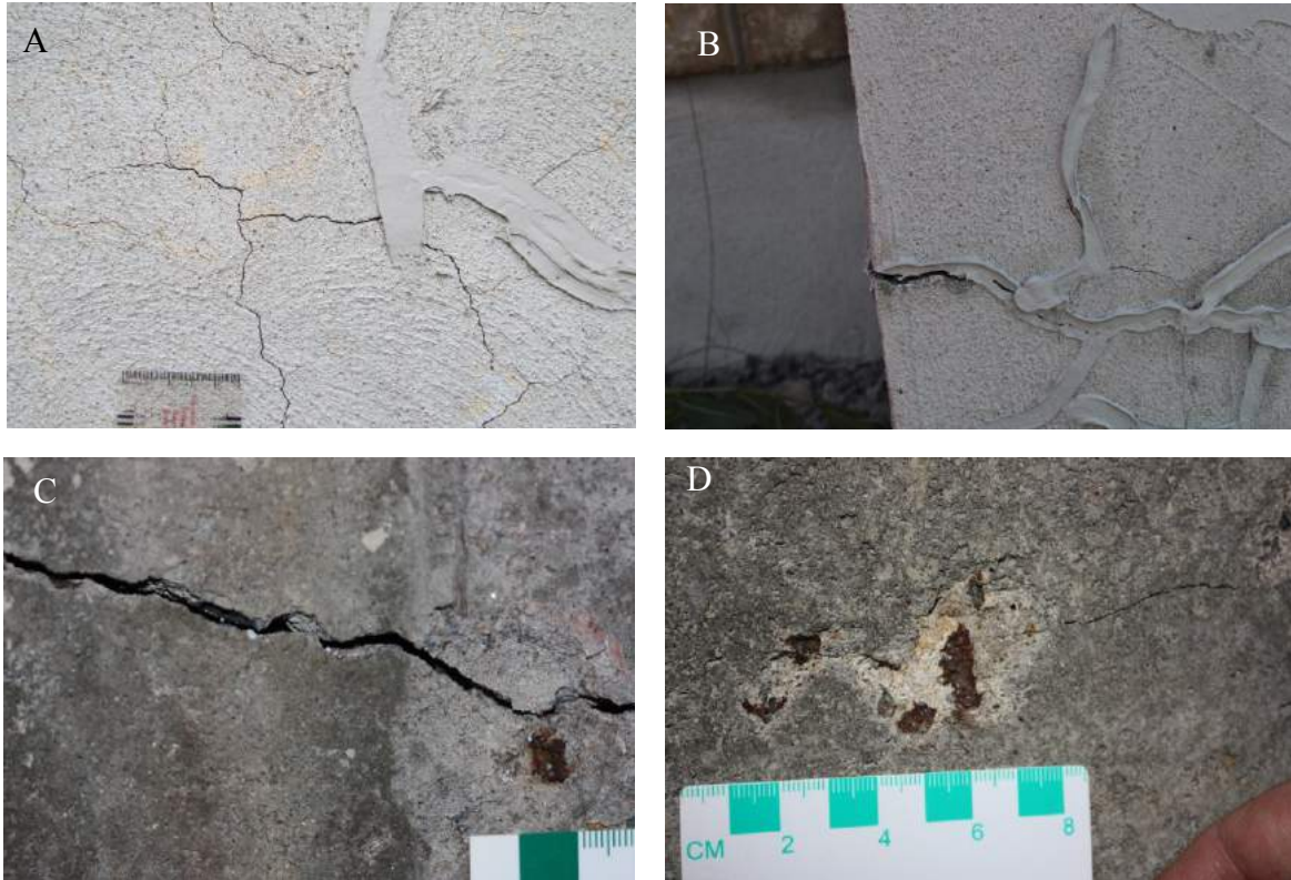
Figure 2: Examples of concrete deterioration features A – Map-cracking in concrete foundation showing some yellowish surface coloration. B – Cracks were filled up with sealant materials to prevent water infiltration. C – Large open cracks seen on the interior side close to an exposed oxidized aggregate particle. D – Pop outs on the interior side of a wall showing oxidized aggregate particles surrounded by whitish secondary products.
