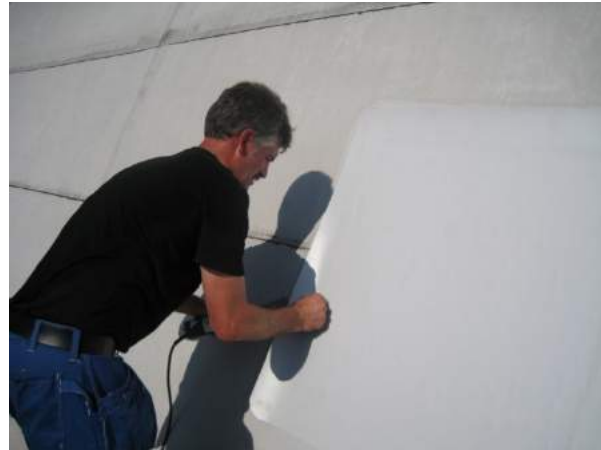
Figure 2: Over-welding the sampling area with a new piece of membrane.
