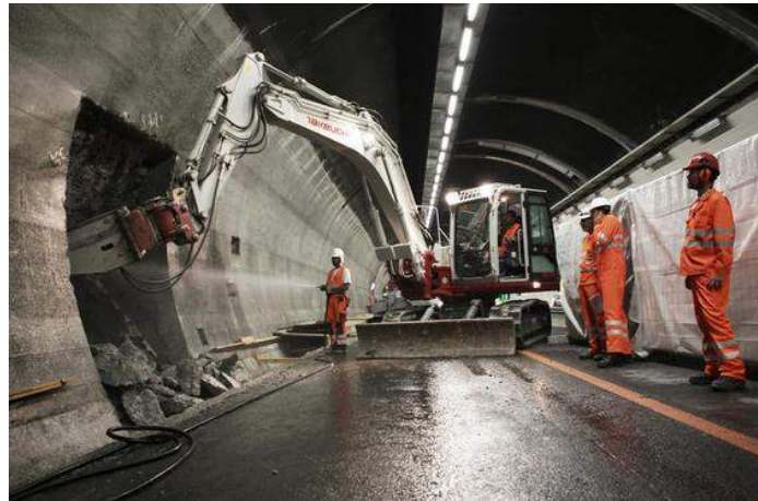
Figure 10: Excavation of escape port in the Reuss- the Reussportport Tunnel.
