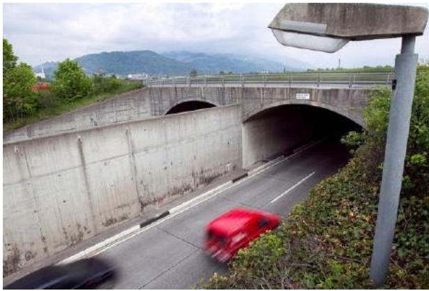
Figure 10: Portal of the Allmend tunnel.
