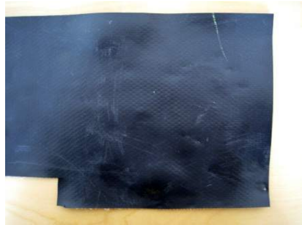
Figure 11: Sample from the Allmend tunnel.
