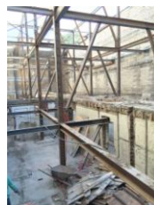
Figure 7. A new steel structural frame, un-veiled as demolition proceeds.
