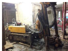
Figure 4. Hydraulic drilling rig installing a set of micropiles.
