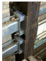
Figure 9. Structural thermal break device detail image.
