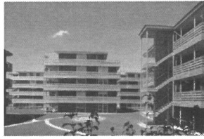
Figure 11 Balance housing development, Fällanden, carcass with visible concrete ceilings and wooden beams at façade level
