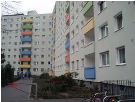
Masonry construction out of hollow-chamber brick
