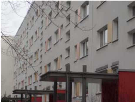
Panelised structure WBS 70
