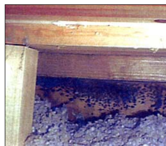
Picture 2 The incidence of condensation and mould growth in the upper, cold corner of cavities in thickly insulated, external, timber-frame walls
