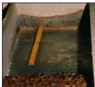
Picture 2 The incidence of condensation and mould growth in the upper, cold corner of cavities in thickly insulated, external, timber-frame walls
