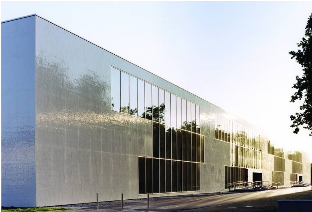
Figure 1 Ventilated rain-screen façade with iridescent glass composite panels (back-side connected) at the GEWOGE, LU-WOGE BASF service centre in Ludwigshafen, Germany. Architects: Allmann Sattler Wappner.
