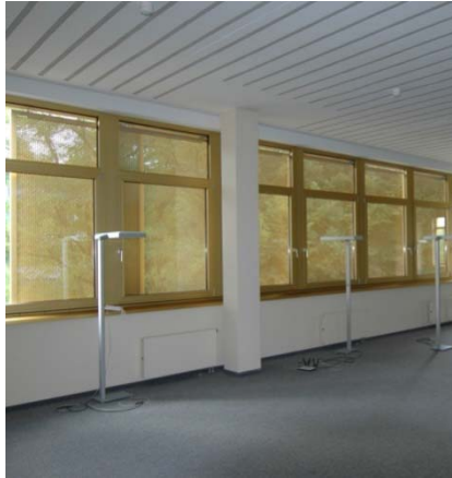
Fig. 7: absorber strips of porous glass installed in thermally active concrete floor in an office room designed for several persons [5] and measured reverberation times with and without absorber strips
