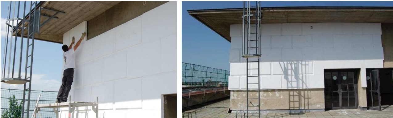
Figure 6: sample area during mounting work and after completion
