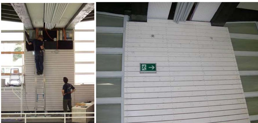
Figure 7: Cameras below the bearings of the main beam - during (left) and after installation (right)
