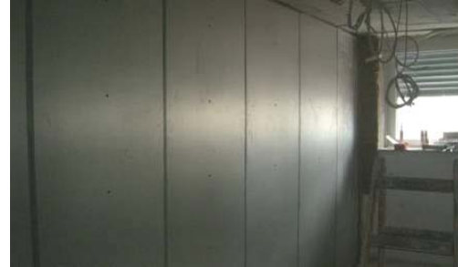
Fig. 7 Positioned panels on the wall surface
