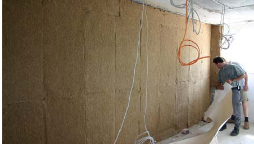
Fig. 6 Hemp fibre insulating mats as an equalising layer
