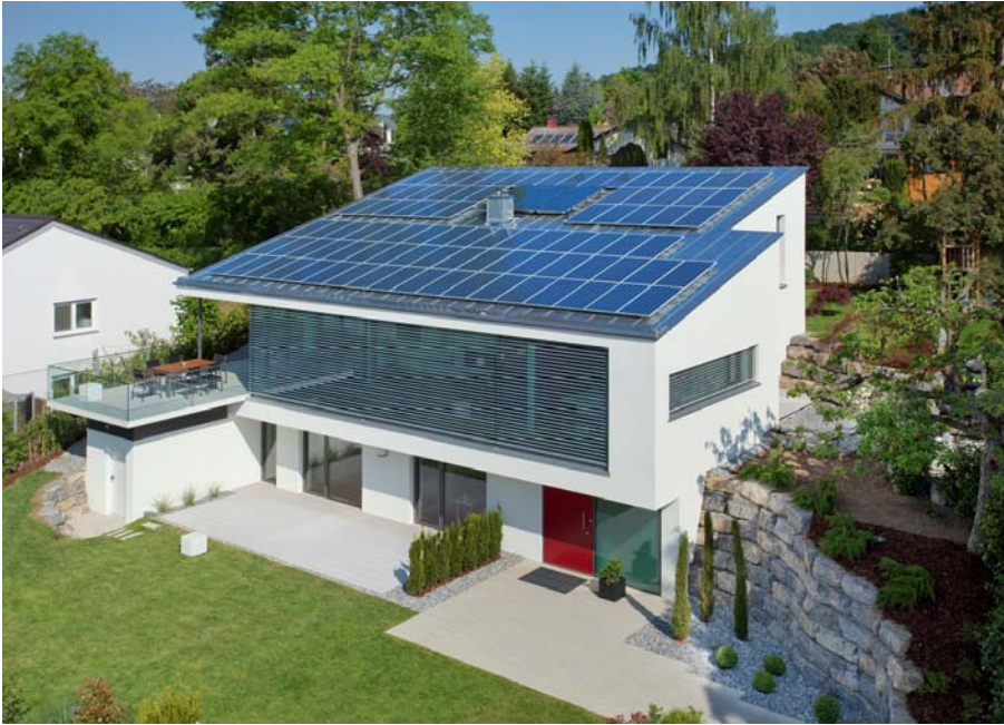
Figure 1: Net-surplus-energy building in Leonberg-Warmbronn Name of the figure: Ansicht.jpg
