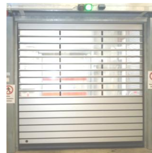
Figure 5: high-speed spiral door
