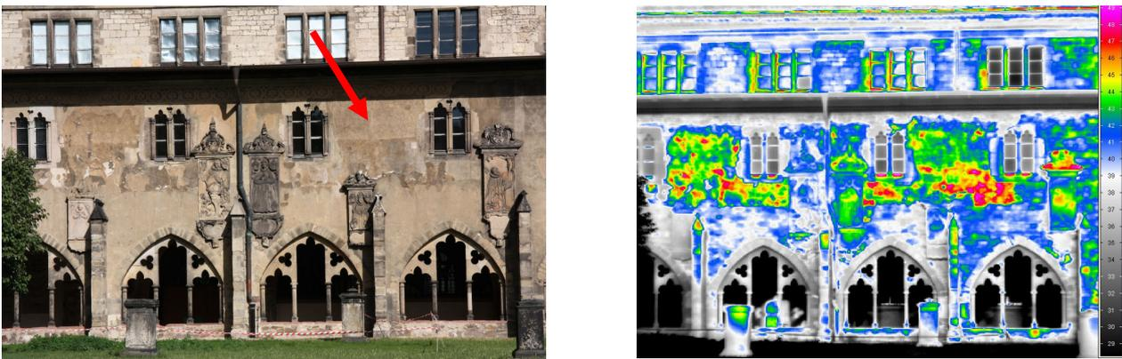
**Fig. 5:** West facade of the cloister of the Cathedral of Magdeburg with the plaster scratches. Left: view of the facade, the arrow indicates the position of the central image. Right: thermogram of the facade after exposed for several hours to sunlight radiation.
